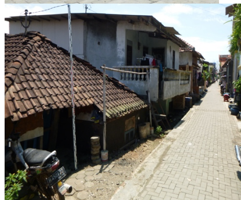
Fig 9: ‘Sinking’ houses Semarang 2018 The roof of the house in the foreground is just 1,20m above street level. The 1th floor balcony of the next house now serves as entrance, while the ground floor serves as basement. (@Julia Illigner).
