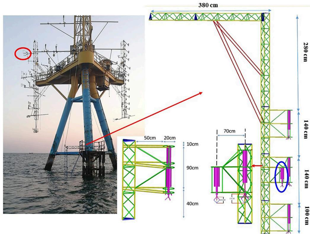
**Figure 1.** Observation platform of the marine meteorology tower in the northern South China Sea (viewed from the north), and the observational framework installed with the ADVs. The instrument highlighted by the red (blue) ellipse is the Campbell Scientific eddy covariance system (Vectrino). ADV, acoustic Doppler velocimetry.
