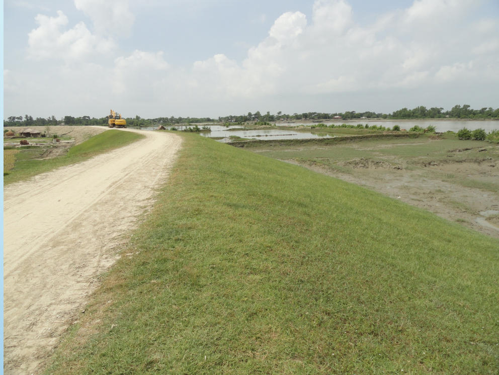
Completed embankment of Polder-33: Year 2021
