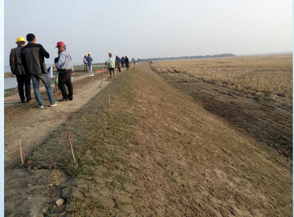
Construction of embankment of Polder-33: Year 2016
