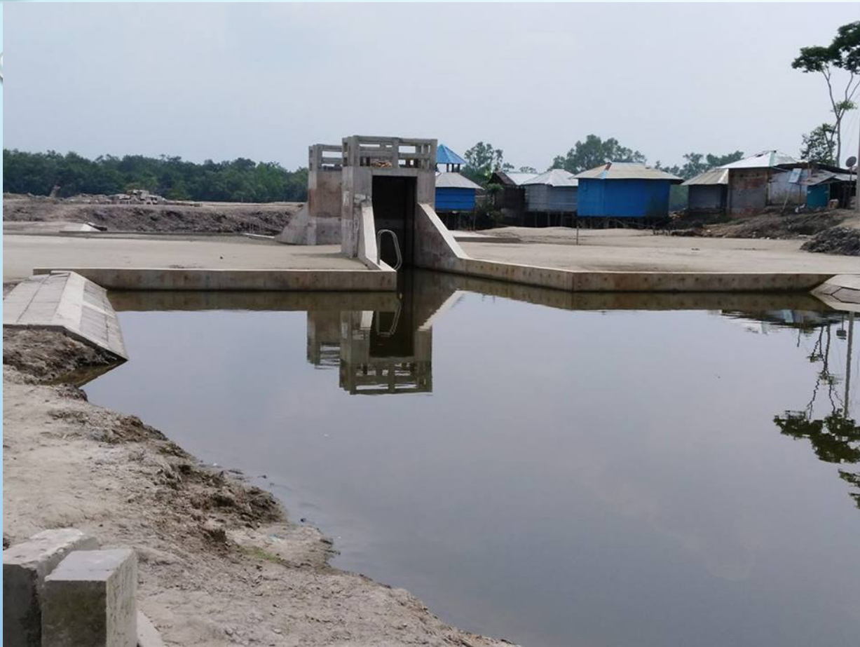
Completed Drainage Structure in Polder-32: Year 2019
